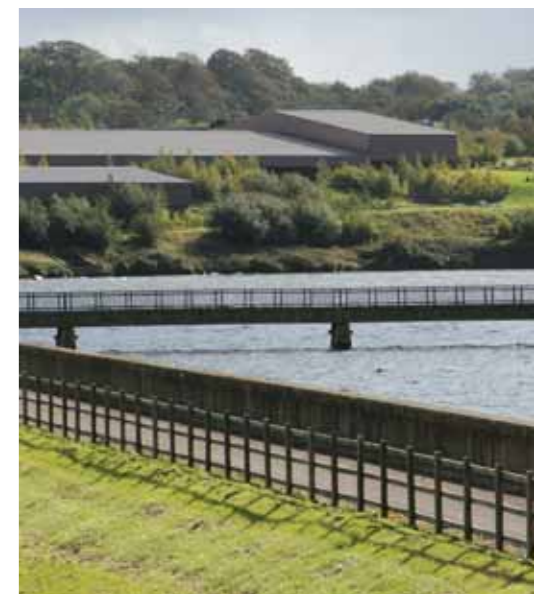
Melbourne Sewage Treatment Works
